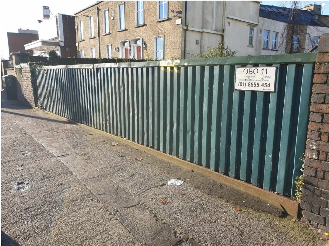
Footpath and east bridge parapet
