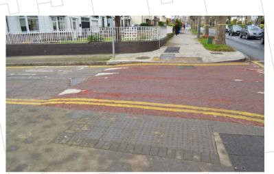
PAVEMENT IN THE ACCESS AREA OF BUSES, SHOULD BE REPAIRED TO PROVIDE AN ADEQUATE HEIGHT OF KNEELING FOR BUSES. LOCATION OF POLES AND LITTERBINS SHOULD GUARANTEE AN ADEQUATE SPACE FOR DISABLED PEOPLE.
