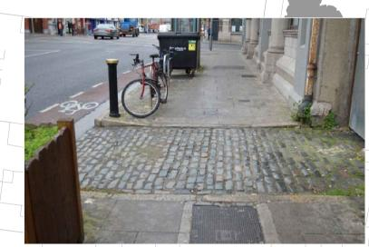
CROSSING POINT AT SIDE ROAD. CHECK VERTICAL DEVIATIONS INFERIOR TO 5 MM. ENSURE A NON-SLIPPERY PAVEMENT
