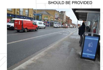
UNCONTROLLED CROSSING POINT WITH ABSENCE OF TACTILE PAVING AND DETERIORATED PAVING IN THE SIDE ROAD. SURFACES SHOULD BE RENOVATED
