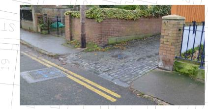
CROSSING POINT AT SIDE ROAD. CHECK VERTICAL DEVIATIONS INFERIOR TO 5 MM. ENSURE A NON-SLIPPERY PAVEMENT.
