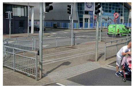
CONTROLLED CROSSING POINT. RED BLISTER TACTILE PAVING SHOULD BE PROVIDED: IN CENTRAL ISLAND. STAGGERED CROSSING TO BE REVIEWED.
