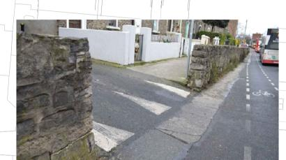
EXCESSIVE GRADIENT AT SIDE ROAD CROSSING WITH THE FOOTPATH. A GRADIENT OF 1:50 MAX. SHOULD BE ENSURED
