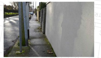
STREET FURNITURE IN FOOTPATH: A MINIMUM WIDTH OF 1200 mm. SHOULD BE ENSURE IN A DISTANCE OF 2000m. LOCATION OF POLES AND LIGHTING COLUMNS SHOULD BE RECONSIDERED. BACK OF THE FOOTPATH OR EDGE BOUNDARY.
