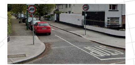
UNCONTROLLED CROSSING POINT. BUFF OR GREY" TACTILE P SHOULD BE CONSIDERED. DEPTH OF 1.2 M, GRADIENT 1:12 MAX. LEVEL DIFFERENCE OF DISHED KERB: 6MM.
