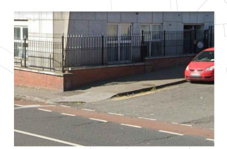
UNCONTROLLED CROSSING. A DISHED KERB AND "BUFF" OR GREY TACTILE PAVING SHOULD BE CONSIDERED DEPTH OF 1.2 M, GRADIENT 1:12 MAX. LEVEL DIFFERENCE OF DISHED KERB: 6MM
