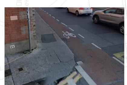
DETERIORATING PAVEMENT IN UNCONTROLLED CROSSING POINT. DISHED KERB TO BE PROVIDED AND "BUFF" OR GREY TACTILE PAVING.
