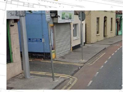
UNCONTROLLED CROSSING POINT AT A SIDE ROAD NO DISHED KERBS AND TACTILE PAVING. A BUFF OR GREY TACTILE PAVING SHOULD BE PROVIDED WITH A WIDTH OF 1.2 m. (3 SLABS)
