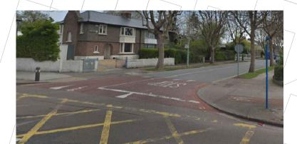
UNCONTROLLED CROSSING POINT. IT SHOULD BE TRATED AS FOR AN IN LINE UNCONTROLLED CROSSING. 1.20 m. WITDH (3 SLABS)
