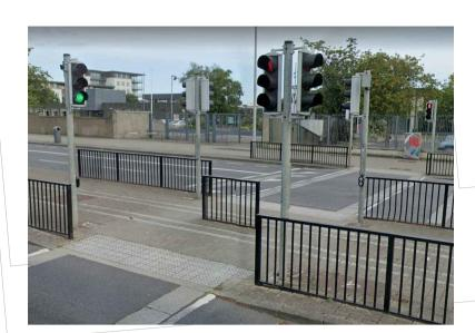
CONTROLLED CROSSING POINT. RED BLISTER TACTILE PAVING SHOULD BE PROVIDED: 0.8m. (2 SLABS). CHECK IF CENTRAL GUARDRAIL IS NECESSARY. (IT IS IN DIRECT LINE OF TRAVEL)
