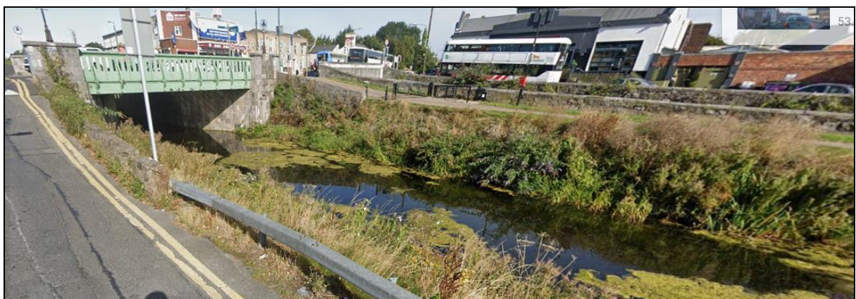
Plate 3: View NE Cross Guns Bridge and canal towards location of R3-CP04 and 07.
